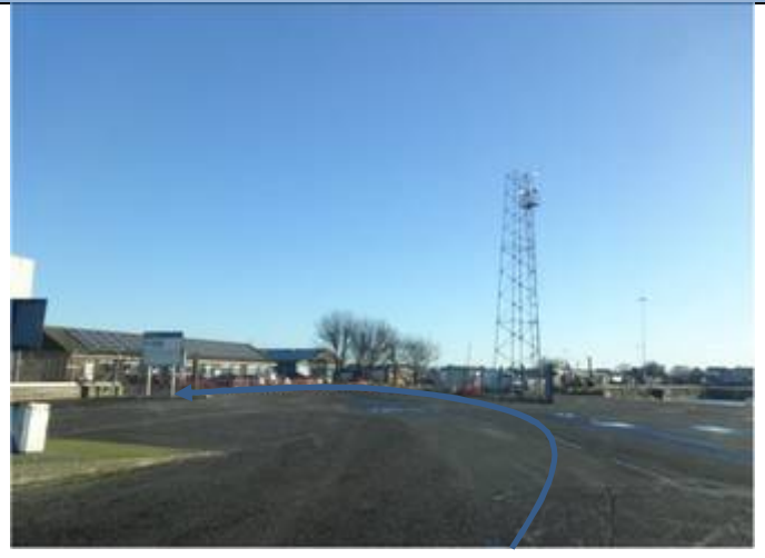
8.4.1.2. – View prior to junction
