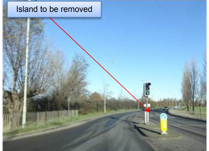
8.4.6.4. – View on junction
