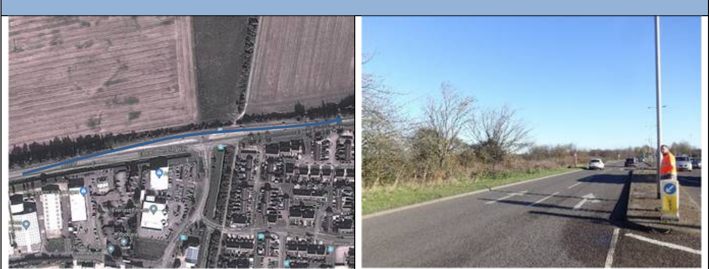
8.5.1.1. – Aerial View of Location 8.5.1.2. – View on left hand bend
