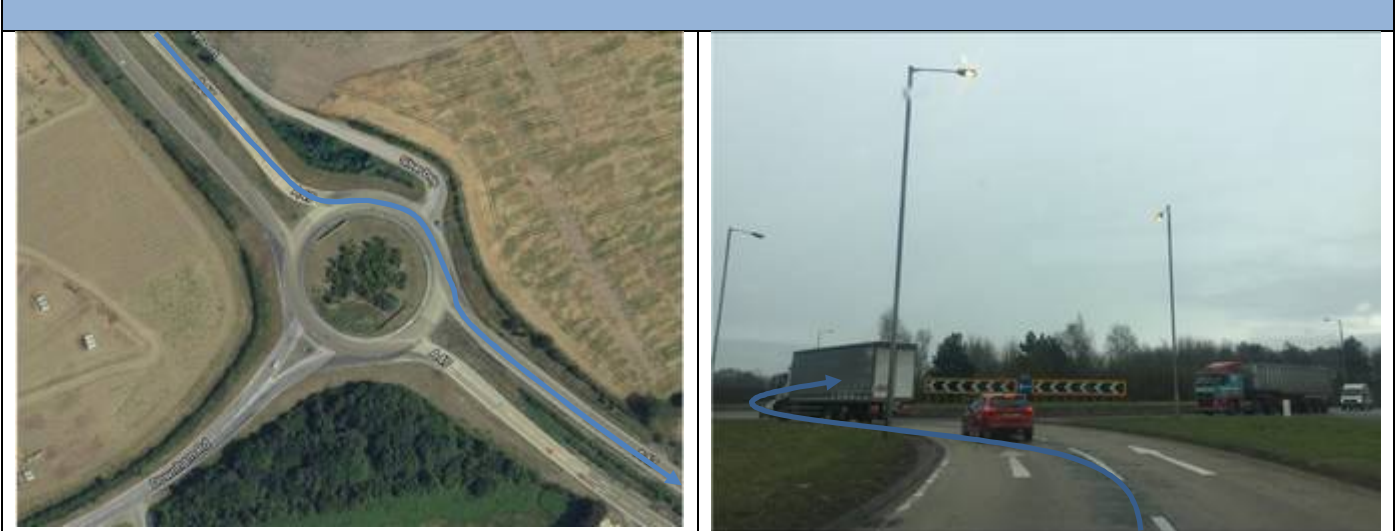
8.8.1.1. – Aerial View of Location 8.8.1.2. – View of entrance to roundabout
