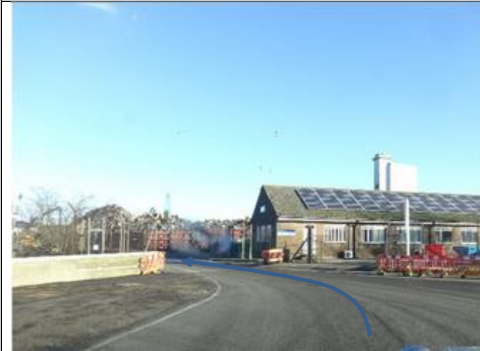
8.4.1.3. – View at crossing
